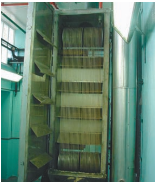
Part of the fuse-fabrication process in India.
